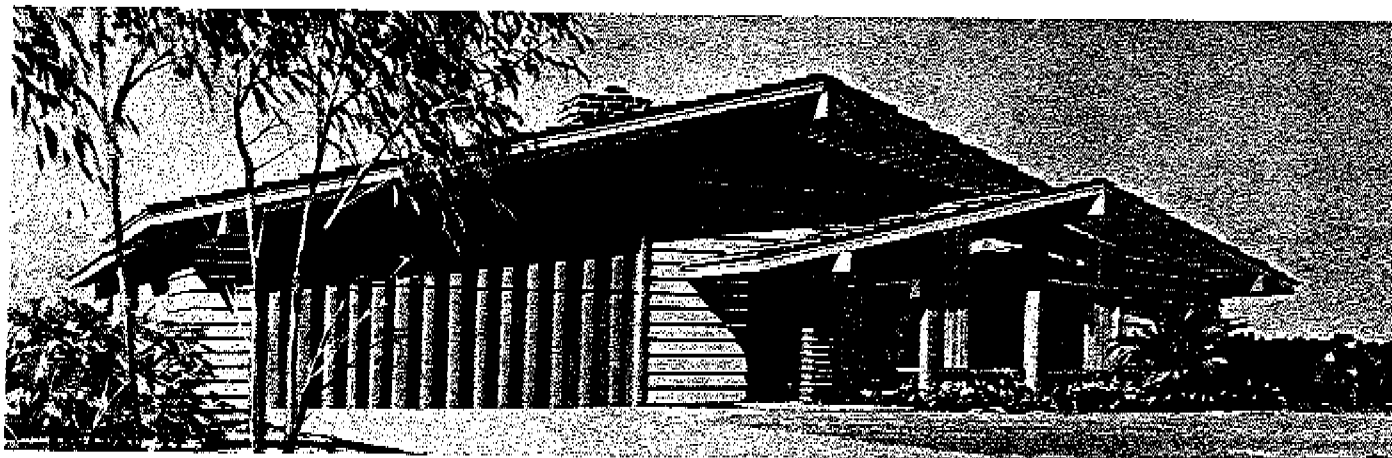
406A —Horizontal and vertical wood siding provides a pleasing contrast to a traditional brick supporting column and chimney.
